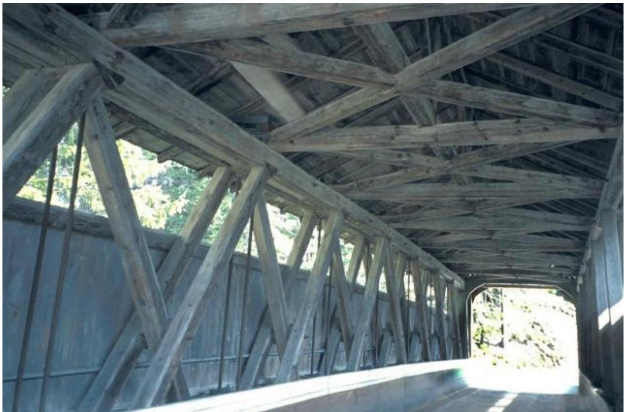
fig. 8: Howe girder system, Graubünden, Switzerland
