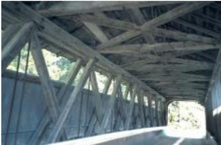
fig. 8: Howe girder system, Graubünden, Switzerland
