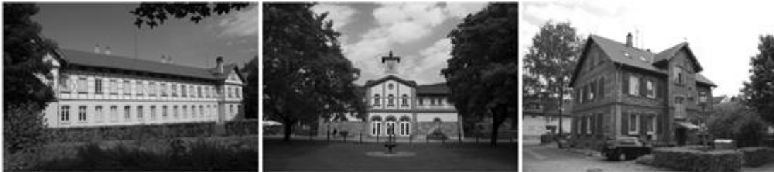
(d) Bleicherstr. 19 backside - built in 1864 (e) Neckarstr. 68 - built in 1869 (f) Bleicherstr. 17 - built in 1886/87
