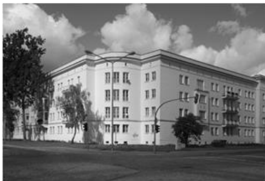
(a) Building in WKII
